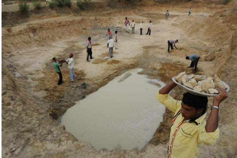
Villagers of Uka at Raghunathpur-II block in Purulia district dig a catchment area for rainwater harvesting. (Samir Jana/HT Photo)
